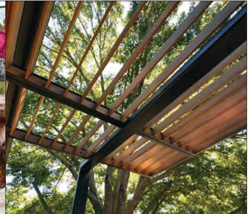
4 Trellis - Black Metal Post and Wood Purlins _____
